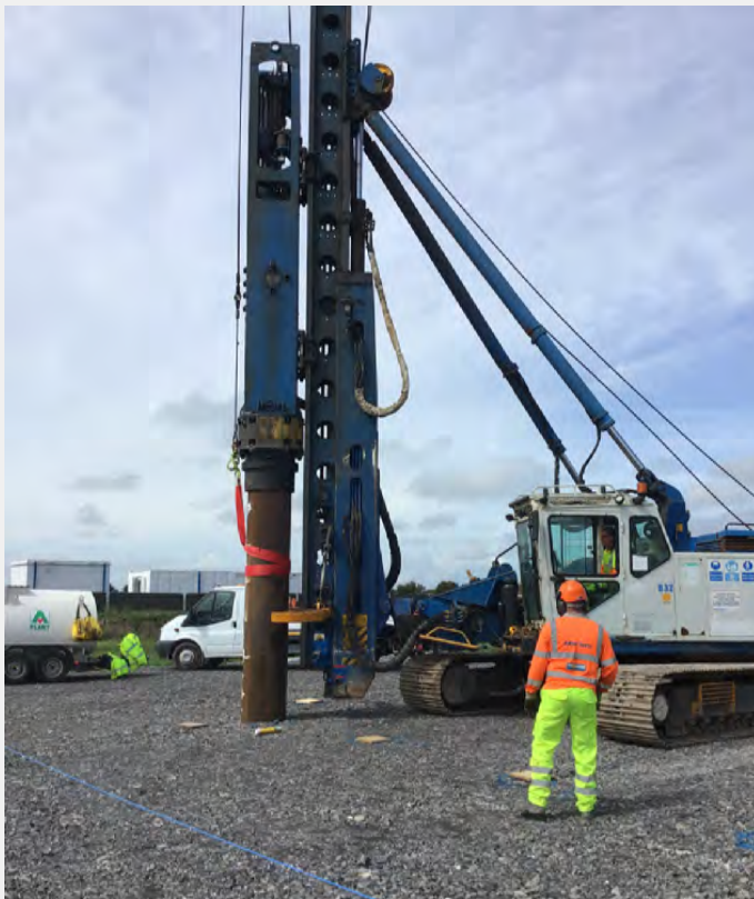
Balfour Beatty's piling rig
