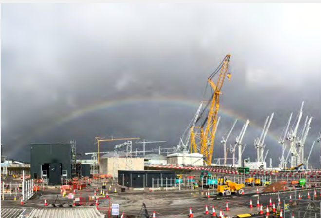
Work is progressing well at Shurton substation
