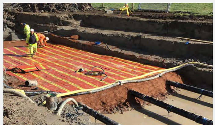
Three cable ducts are laid in each trench
